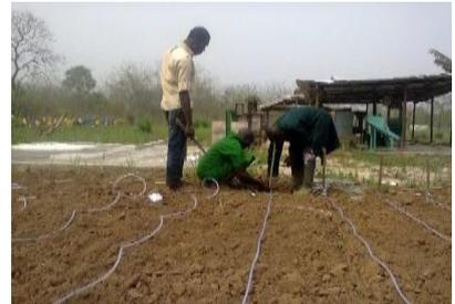
Plate 2: Installation Layout of the IDI system
