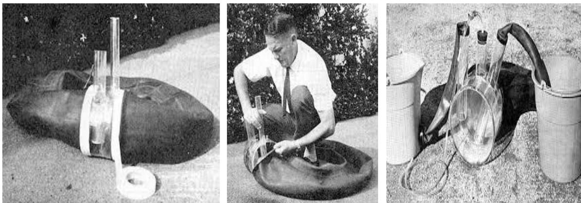
Figure 4. Innertube Digester; Methane Digesters for Fuel Gas and Fertilizer (Fry *et al.*, 1973)
