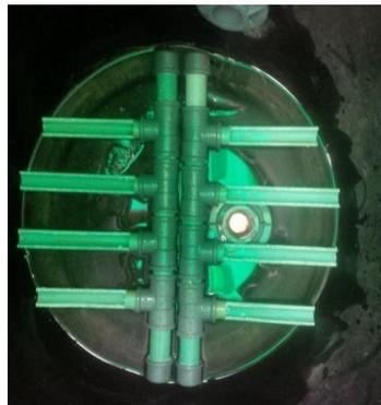
**Figure 2:** Manifolds with Lateral Pipes
