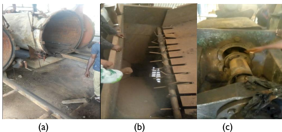
Figure 1. Abandoned Facilities (a) Sterilizer (b) Stripper (c) Digester Screw Press
